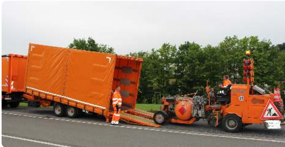
Quick and easy loading of a road marking machine: machine is automatically locked and secured by a coupling after the ascent at the front wall
